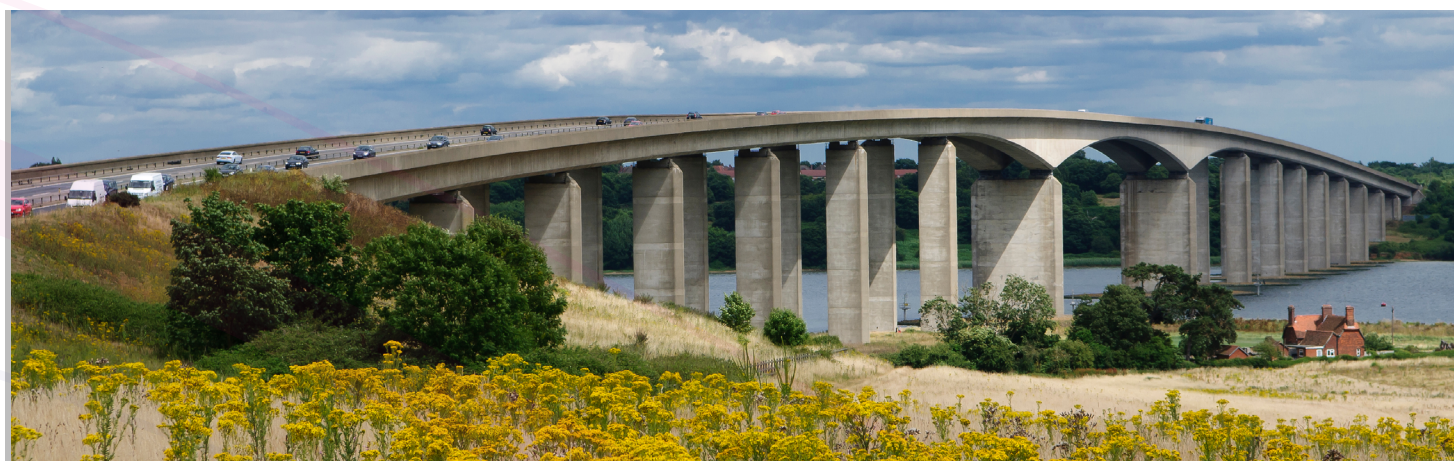
The Orwell Bridge in Ipswich
